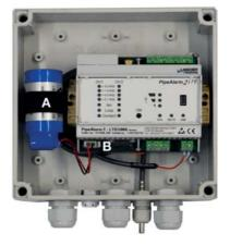
Click the mount and the new battery (**A**) into place on the top-hat rail. Attach the polarity-reversal-protected battery connector (**B**) of the new battery (LANCI-ER Monitoring order number 075969.000) to the X6 connector (see page 6).
