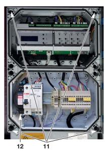
Attach the PipeMonitor housing firmly to the wall using the 4 outer drill holes (11).
