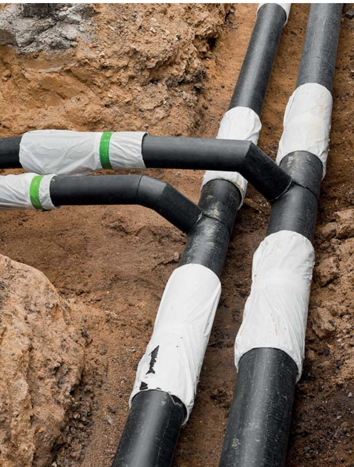
Surveillance pair arrangements in insulated sheath pipe systems for district heating
