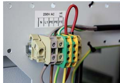
Figure: terminal configuration at delivery of a complete system in a closet; top terminal input: external power supply.
